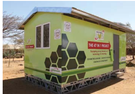
A container constructed from prefabricated recycled ('green') materials, fully equipped with a solar-powered server and 10 solar-powered computers.
